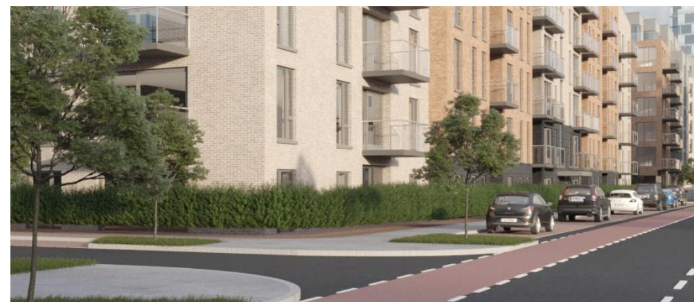
Threshold Condition 1 example on, Block 11
