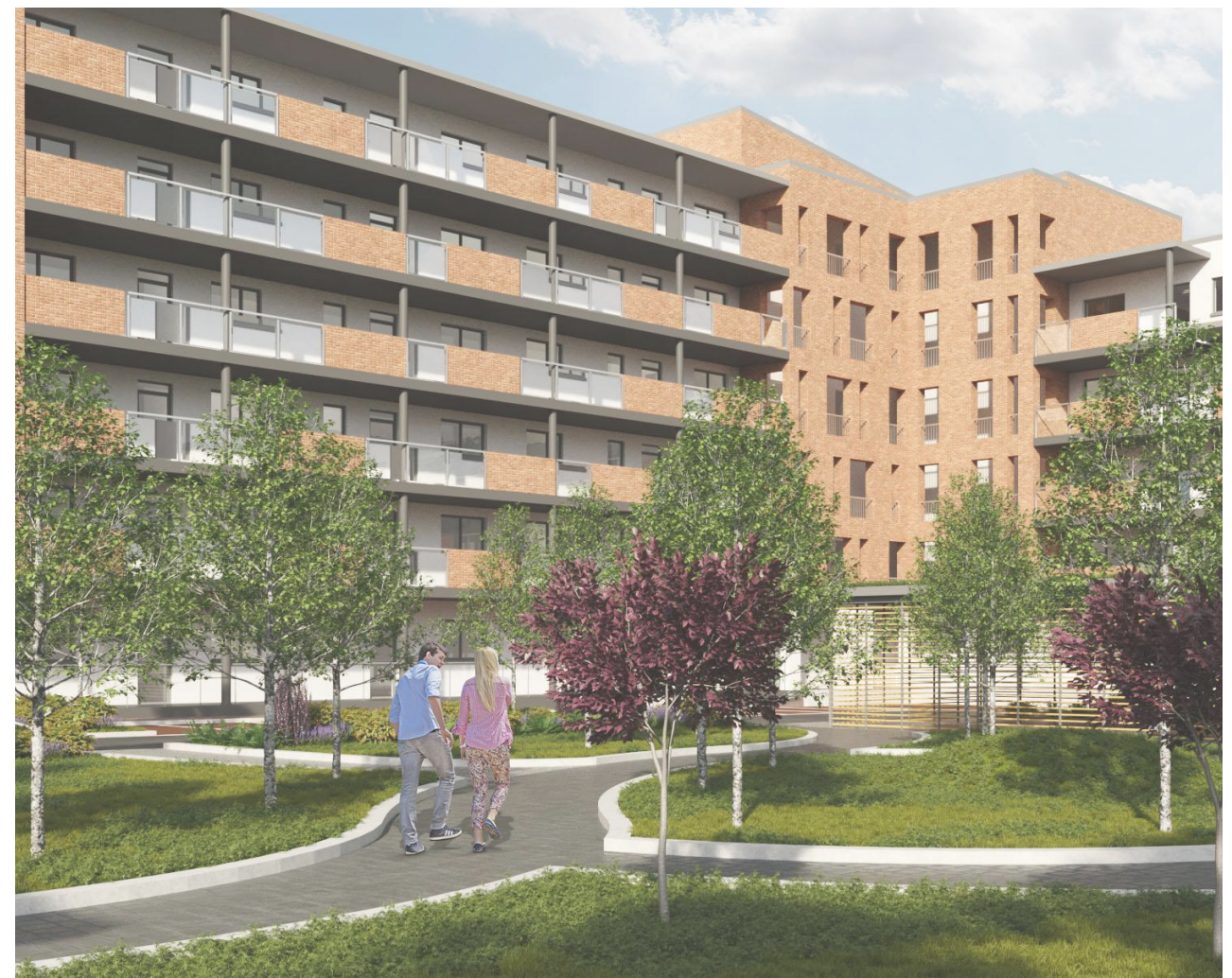
View of Block 11 from east with landscaped communal open space in foreground
